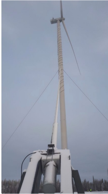
Figure 2-4: Cable-stayed tower for Vestas V150-4.2 MW as installed and operated in the Viinamäki wind farm in Finland. Reproduced from [WFBOP].
